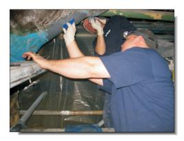
office building in lower Manhattan, developed a leak where the line joined the main header running just under the ceiling.
