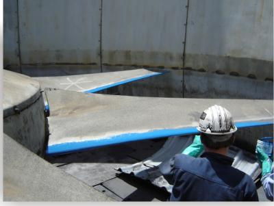
This coal fired power station located in Western Australia was experiencing erosion on their fiberglass cooling tower fan blades. The ash in the air was causing accelerated wear on the leading edges.
