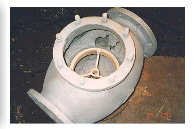
This sea water valve from a ZIM Line vessel was desperately in need of replacement. However, these valves were not available any more and "replacement" was no longer a viable solution.
