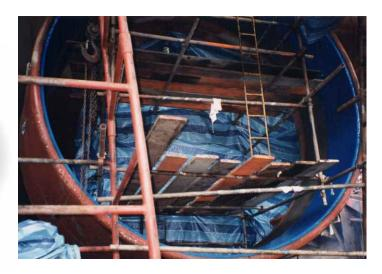
These photos illustrate the very successful application of DuraTough DP & DL to a pair of large KORT Nozzles on the O/MV Mighty Servant 2.
