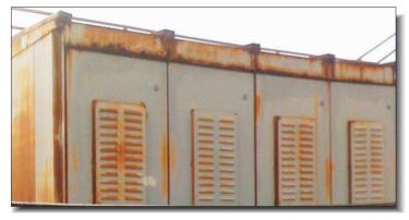
These electrical cabinets at a sewage treatment plant in Tennessee were severely corroded and needed immediate remedial work. The plant engineers wanted a surface tolerant, corrosion protection coating system with minimal V.O.C. issues.
