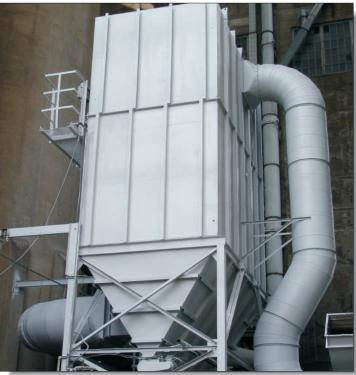
The conventional paint system on this dust collection equipment located at a large grain processing plant in Quebec had failed and was no longer providing corrosion protection to the steelwork. The plant's maintenance engineers were looking for a high performance, corrosion resistant coating system that did not require grit blasting prior to its application.
