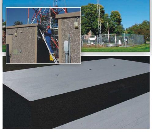
This weather station, located in the Mid Atlantic Region, had serious leaking problems through the concrete roofs which were affecting the sensitive electronic weather monitoring equipment located in these pre-fabricated buildings. The existing roof coating had failed and water was
