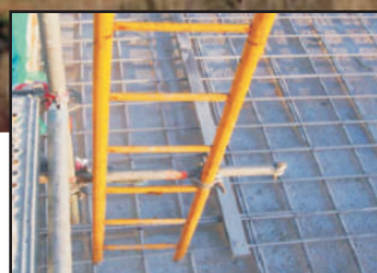
SuperBond Sprayed Over Existing Concrete & Reinforcing Bar.
