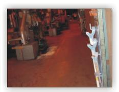
The existing floor coatings at this Australian power station were badly deteriorated and needed to be replaced. The plant engineers wanted a high performance floor protection system that would give them better results than the previous conventional paint system that had been used.
