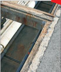
It was suggested that all of the loose material in the damaged areas surrounding the access plates be removed and then cleaned. **ENECRETE DuraQuartz** was then used to build up and level out the damaged concrete surfaces.
