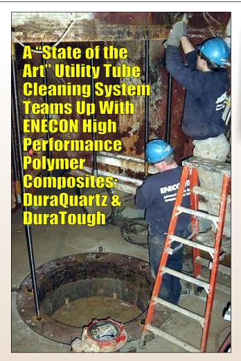
A large power station on Long Island, New York, opted to install a highly specialized tube cleaning system manufactured in Germany to keep its main condensers running at peak efficiency. However, the limited space available required custom design and fabrication of support piping "spool" pieces to anchor the equipment and tie the unit into the
