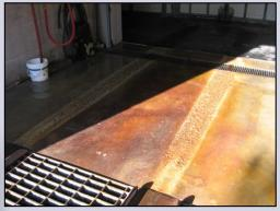
The parking area for the Zamboni machine used to groom the ice at an ice rink at a New Jersey prep school was severely damaged from a combination of melting ice and the studded tires on the Zamboni machine.
