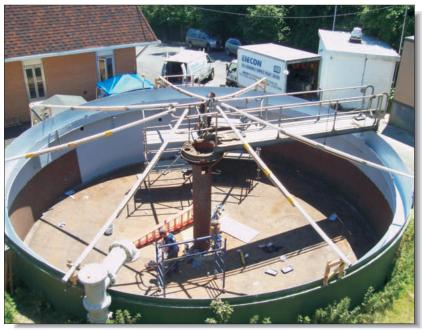
This 40 year old steel influent sewage tank located at a waste water treatment facility in the Northeastern U.S. was suffering from severe corrosion.
