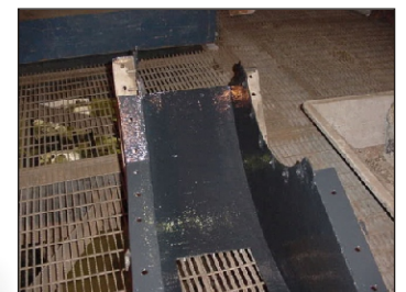
Two coats of CHEMCLADSC were applied to all interior surfaces and flanges.
