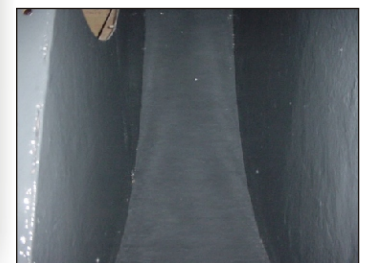
Two coats of CHEMCLADSC were applied to all interior surfaces and flanges.
