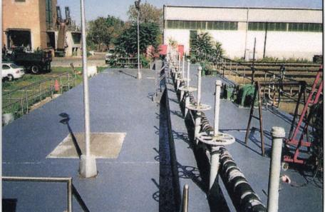
system. Under the watchful eyes of ENECON North East's Field Engineering Team, all cracks in the concrete decks were first repaired with ENECRETE DuraQuartz and then the entire area was protected with CHEMCLAD SC.
