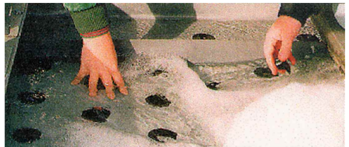
Problems solved & pans protected with CHEMCLAD SC.
