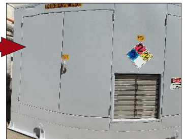
Electrical cabinet. Prepared by pressure washing then two coats of ENESEAL® CR.
