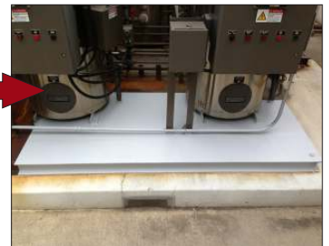
Chemical treatment process station base. Prepared by pressure washing then two coats of ENESEAL® CR.
