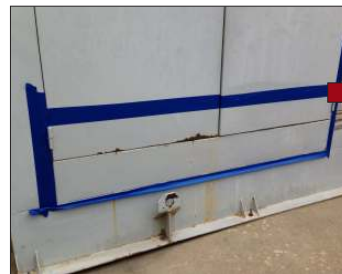
Electrical cabinet. Prepared by pressure washing then two coats of ENESEAL® CR.
