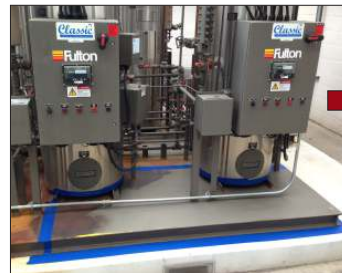
Chemical treatment process station base. Prepared by pressure washing then two coats of ENESEAL® CR.
