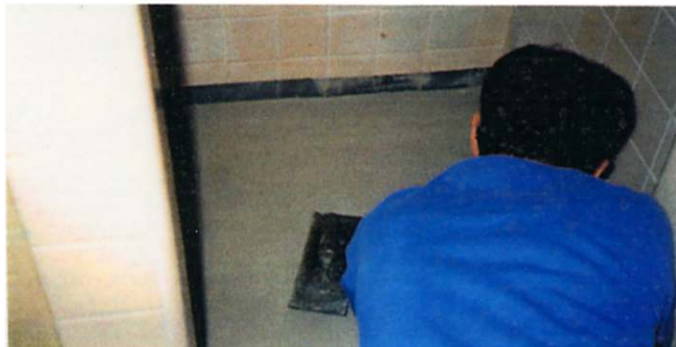
A simple trowel is all that's needed to apply DuraQuartz.
