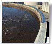
The steel plating on this clarifier tank rim, which serves as a track for the tank's scraping bridge wheels, had been in service for 15 years. Located at a Southern Louisiana wastewater treatment facility, the bridge makes approximately one full rotation every minute.
