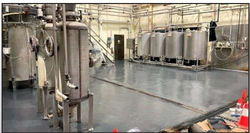
Years of constant acid attack on this 40-year-old floor at a juice processing plant in Pennsylvania caused severe erosion damage to the concrete. The local ENECON District Sales Manager was called in to provide a solution.
