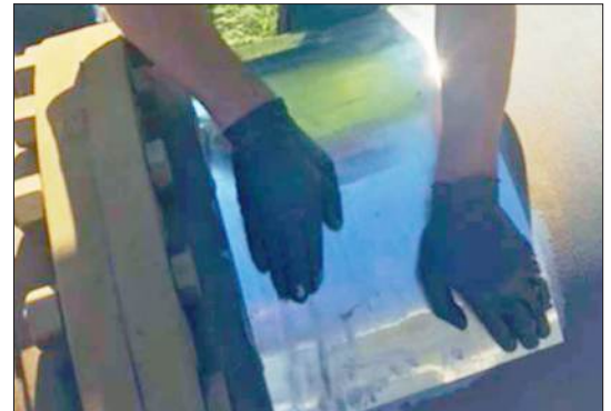
Bonding the stainless steel plate
