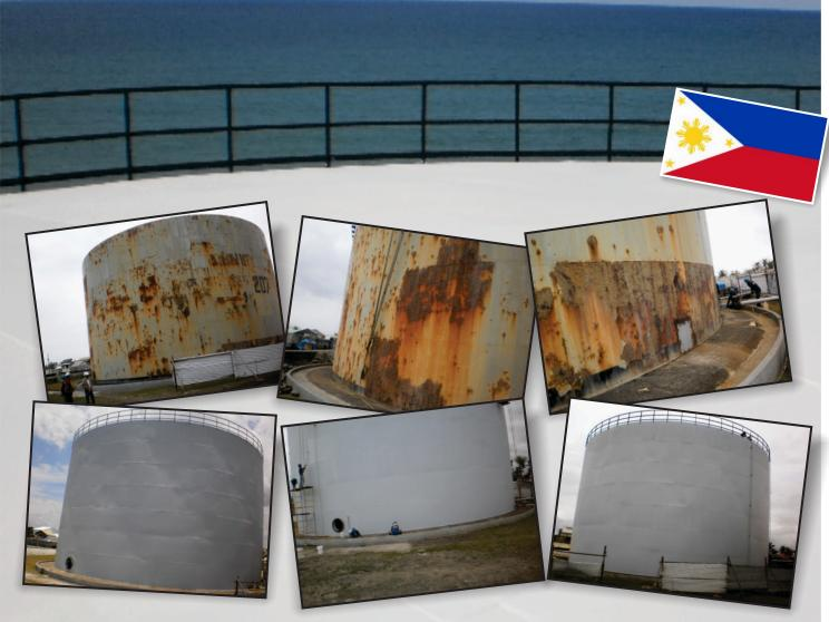
This large gasoline tank located at one of the largest oil companies in the Philippines had been suffering from severe corrosion.
